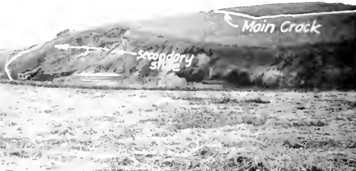
These pictures show volume and force developed by a circular type slide, such as occurred at Kellogg Hills
